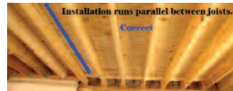
Figure 1 shows how an in-ceiling screen (blue line) should be attached parallel to the ceiling joists and in between them. This is a strong and structurally sound installation.
